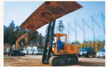
Lifting laying iron plate
